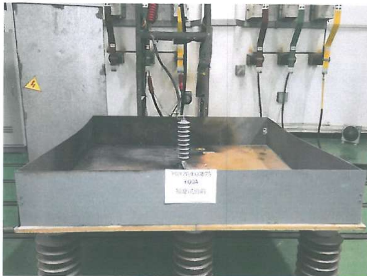
5# Arrester before short-circuit test (600A)
