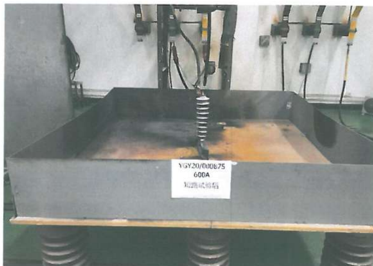
5# Arrester after short-circuit test (600A)
